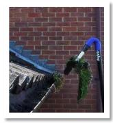
away from gutter then switch vacuum motors off, releasing grass from the tool. IMPORTANT stand to the side when doing this and ensure you can drop the grass **safely** to the ground before releasing the tuft.
